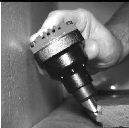
Use the PowerPalm nailer on the last couple of finishing rows, starter rows, end-strips or transitions.
