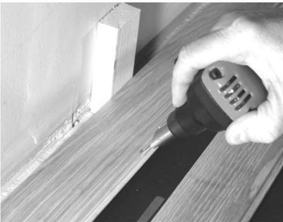
Use the PowerPalm nailer to nail down your starter rows. Be sure to leave the recommended expansion space between the wall and your starter rows. Use the PowerPalm for 2-3 rows or until you are far enough from the wall to start using a Powernailer®.
